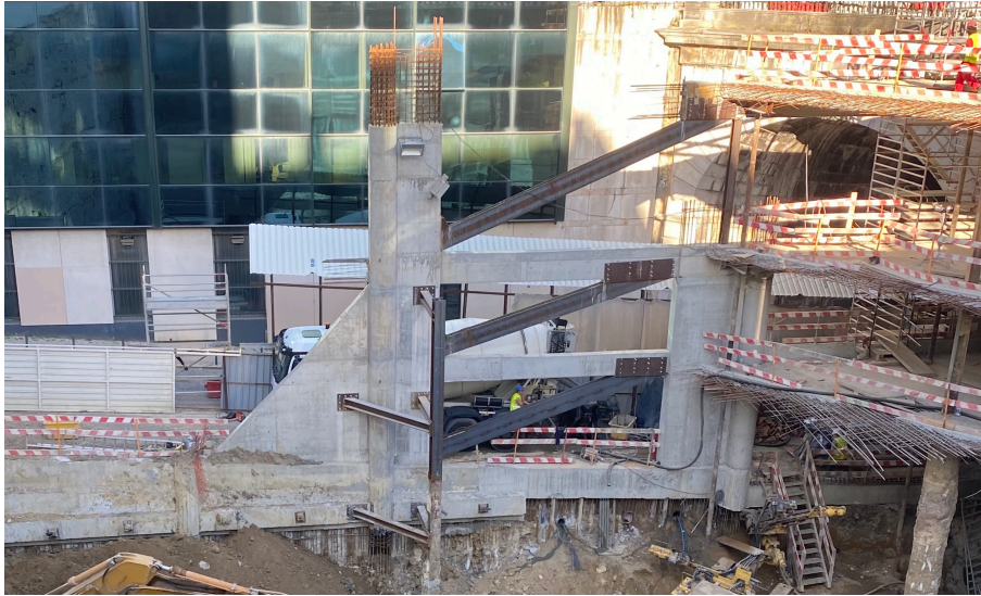
Figure 4 – Alignment A-B – Reaction frame
