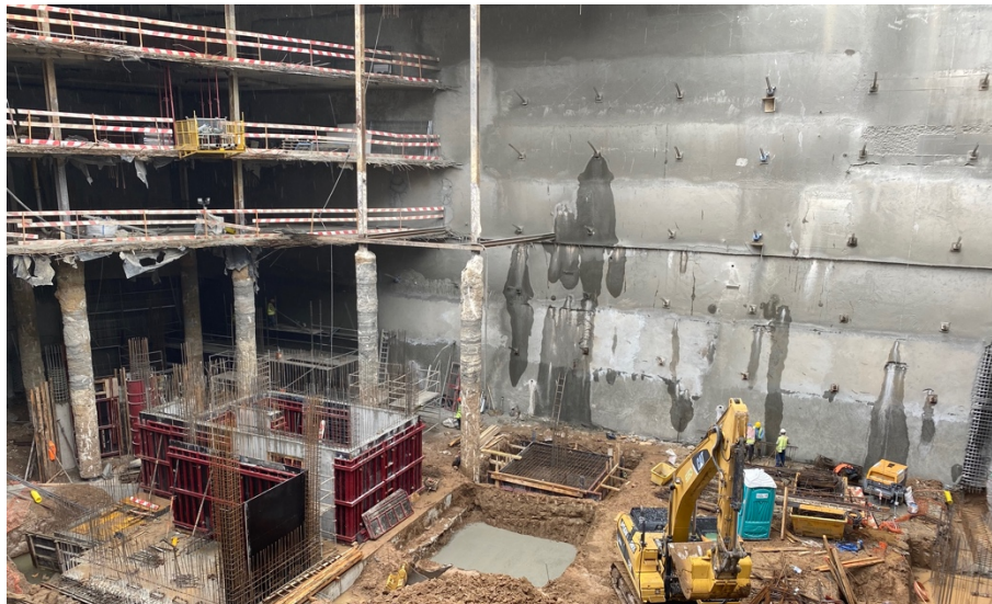
Figure 6 – View of the excavation at the final level
